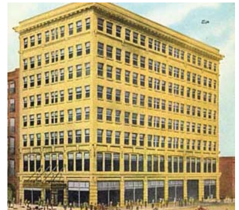
The Pence Automobile Company (shown here on a 1910 postcard) exemplifies the phenomenal growth of the auto trade during the early 20th century. The Classical Revival-style building, designed by Long and Long of Minneapolis, had floors devoted to sales showrooms and offices; automobile assembly, finishing, repair and service; and storage for parts, accessories and completed vehicles.
