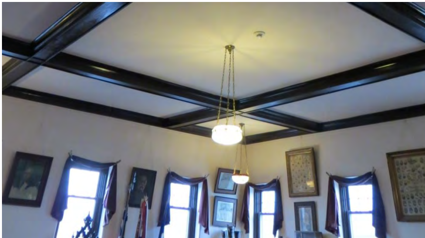
PHOTO 0001: Existing ceiling plaster w/wood box beams
