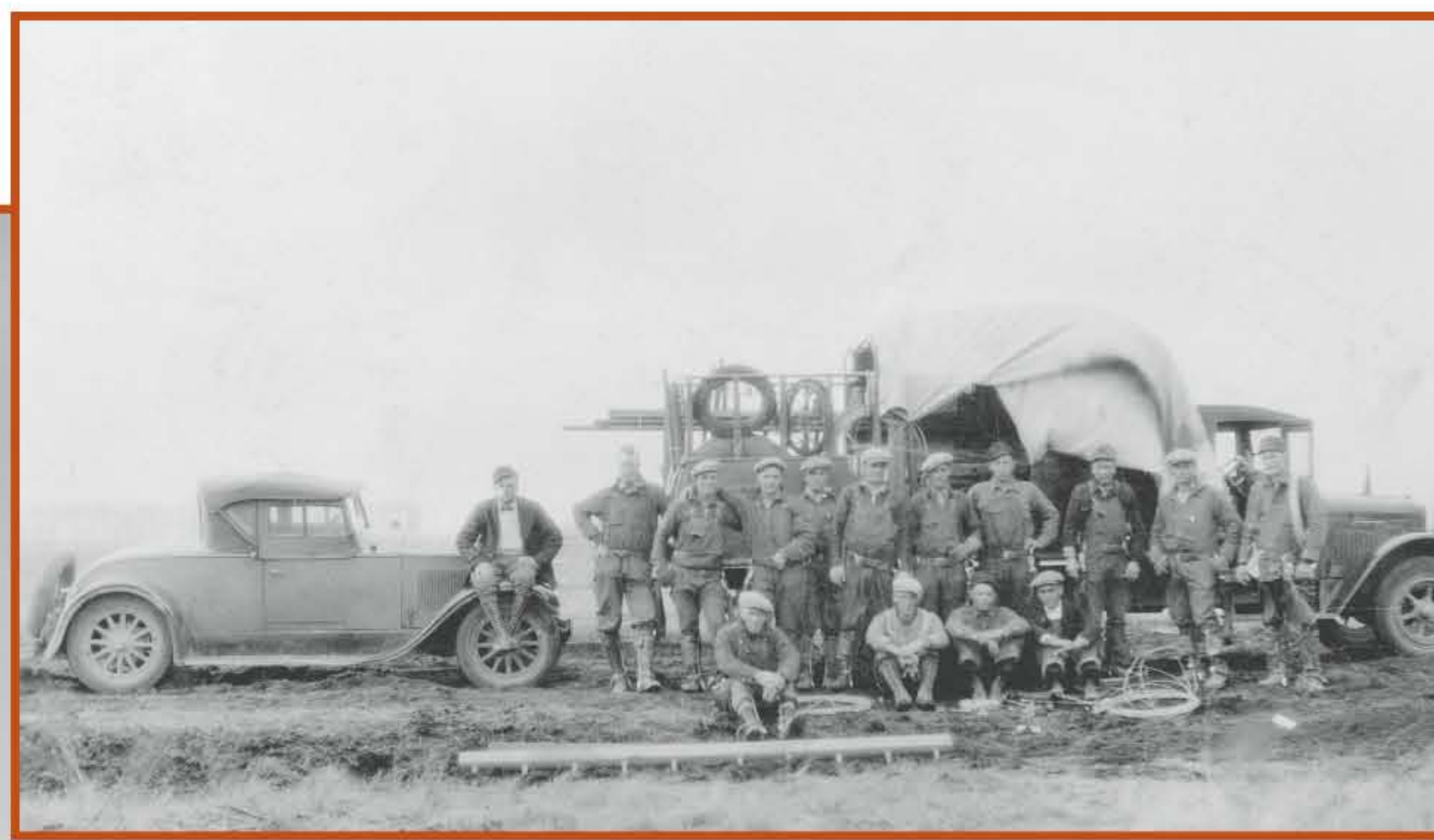
REA line crew, Iron Range, 1930s. Less than 13% of Minnesota farms had electricity in the 1930s. By 1939, the number grew to 30%
