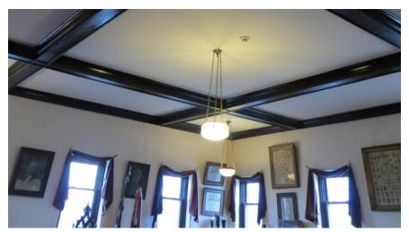
LABELED PHOTO EXAMPLE: PHOTO 0001: Existing ceiling plaster w/wood box beams
