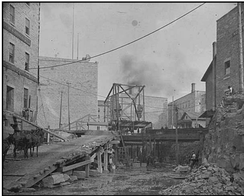
Working on the West Side canal (Minnesota Historical Society)
