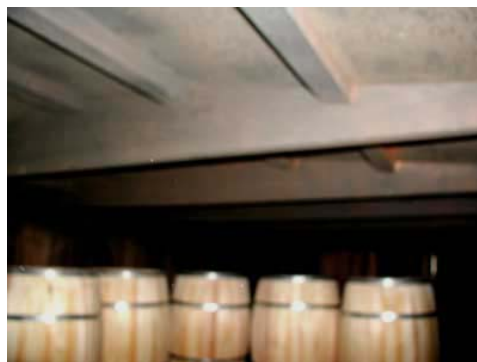
Figure 5: Interior view of the ceiling.
