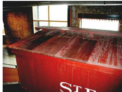
Figure 11: Overview of roof repairs.
