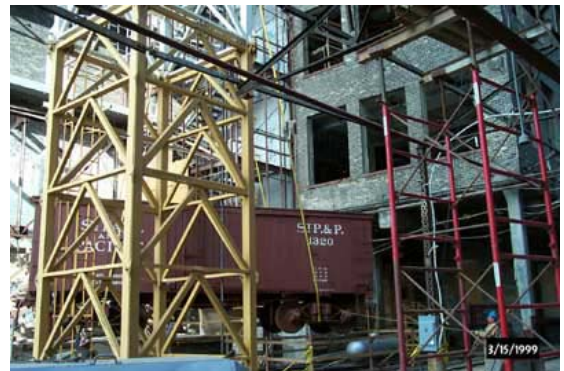
Figure 2: Moving the box car into the Mill City Museum Rail Corridor area.
