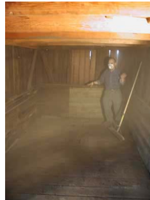
Figure 4: Cleaning of interior in progress.
