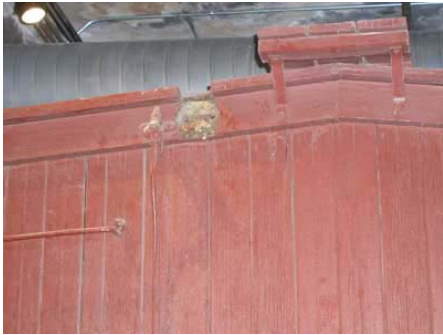
Figure 16: Before treatment view showing brake mechanism attachment area.
