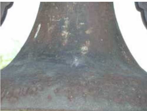
Figure 4: Detail of exterior bell surface before treatment showing corrosion, weather metal, and organic deposits.
