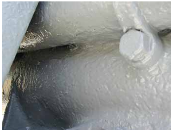
Figure 14. PR recoil tube area after epoxy fills and paint.
