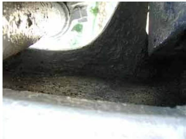
Figure 12. Underside of the swivel mount showing rust stabilizer application.
