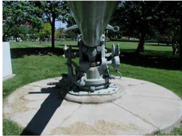
Figure 4. The front underside area of the gun before treatment. Note the rust stains near the bolts on the concrete support base.
