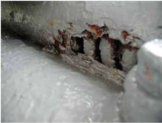
Figure 13. PR side recoil tube springs exposed due to loss from corrosion.
